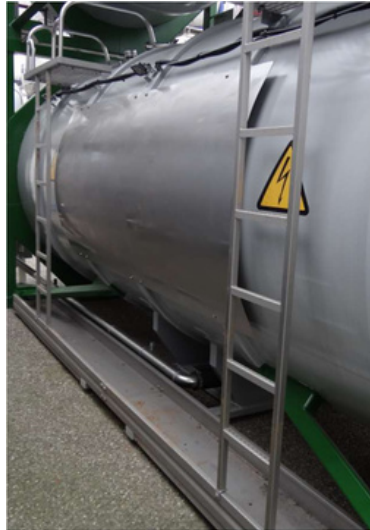
Figure 5: 2 sets of ladders for tank top access
